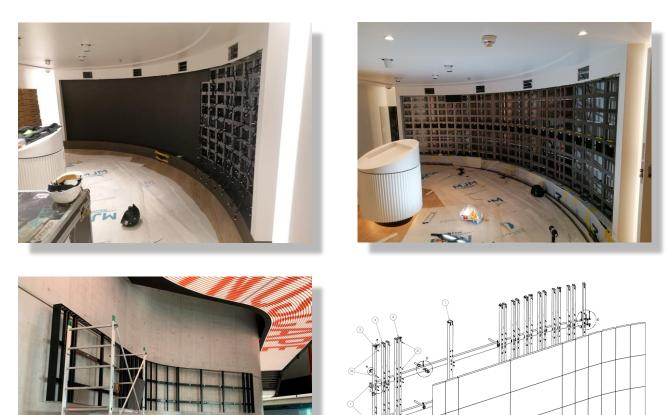
OMB has special skills in the development and production of LED mounting structures for curved walls.
